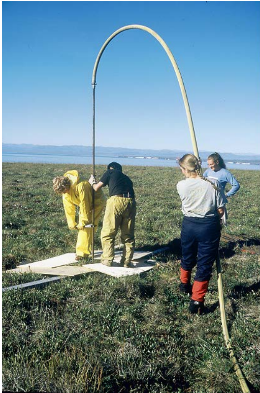
Installation of ground temperature cable, Herschel Island
