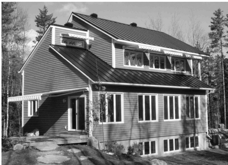
Figure 8: The EcoTerra house, showing retractable awnings above the upper windows.
