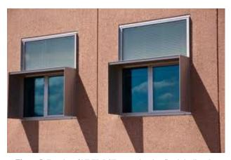
**Figure 5:** Exterior of NREL RSF space showing fixed shading (lower portion) and light louvers (upper portion).
