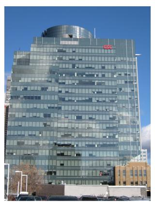
**Figure 2:** Typical shade deployment levels of a south-west facing office building façade in the winter.
