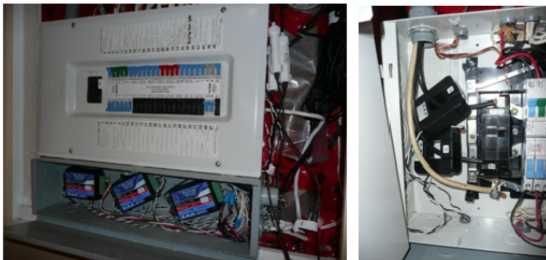
Figure 3.2: Measuring devices installed at the electric panel of a participant in the electric measurement project.
