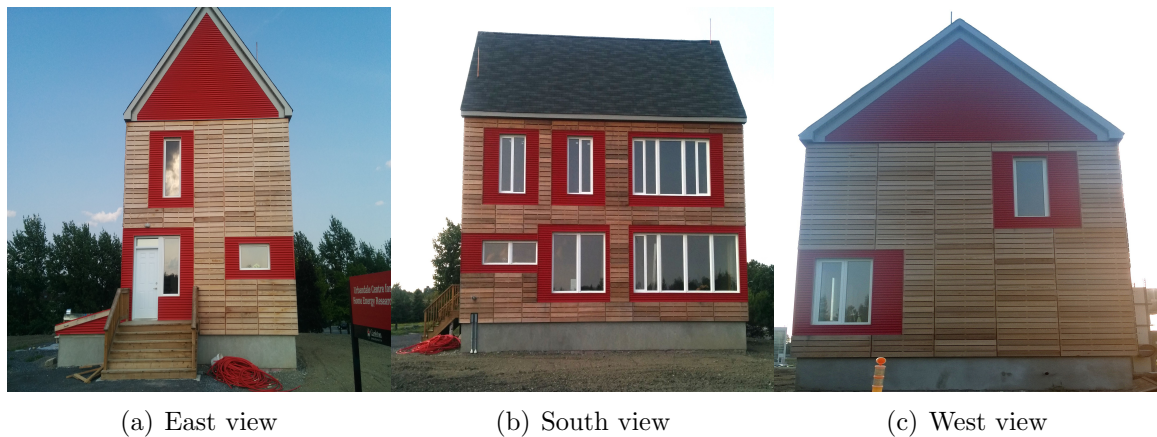
Figure 2.9: Urbandale CHEeR house, showing window positions
