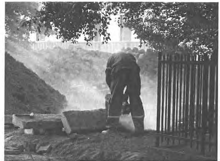
Figure 8.8 Chłodna Street under construction. Warsaw, 2010.
