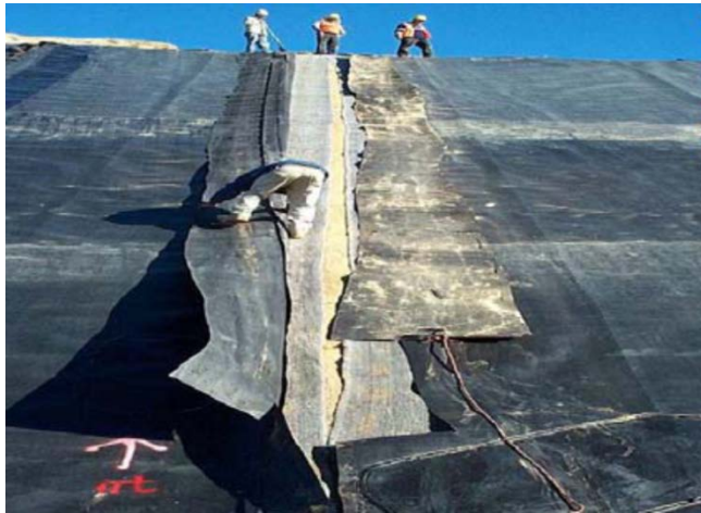
GCL panel shrinkage in California, Thiel et al., 2005
