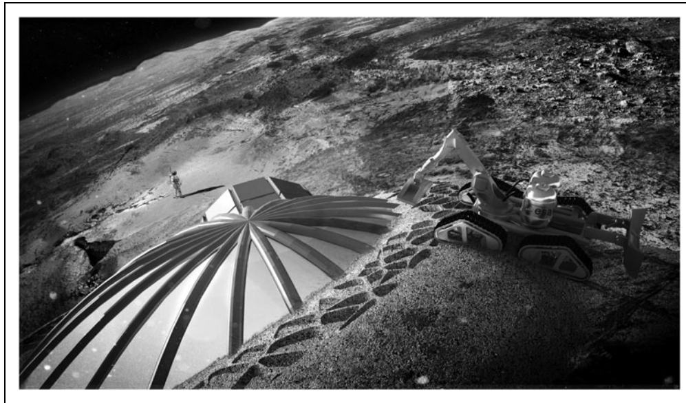
Fig. 4. Mobile rovers 3D printing regolith on the Moon [credit European Space Agency].
