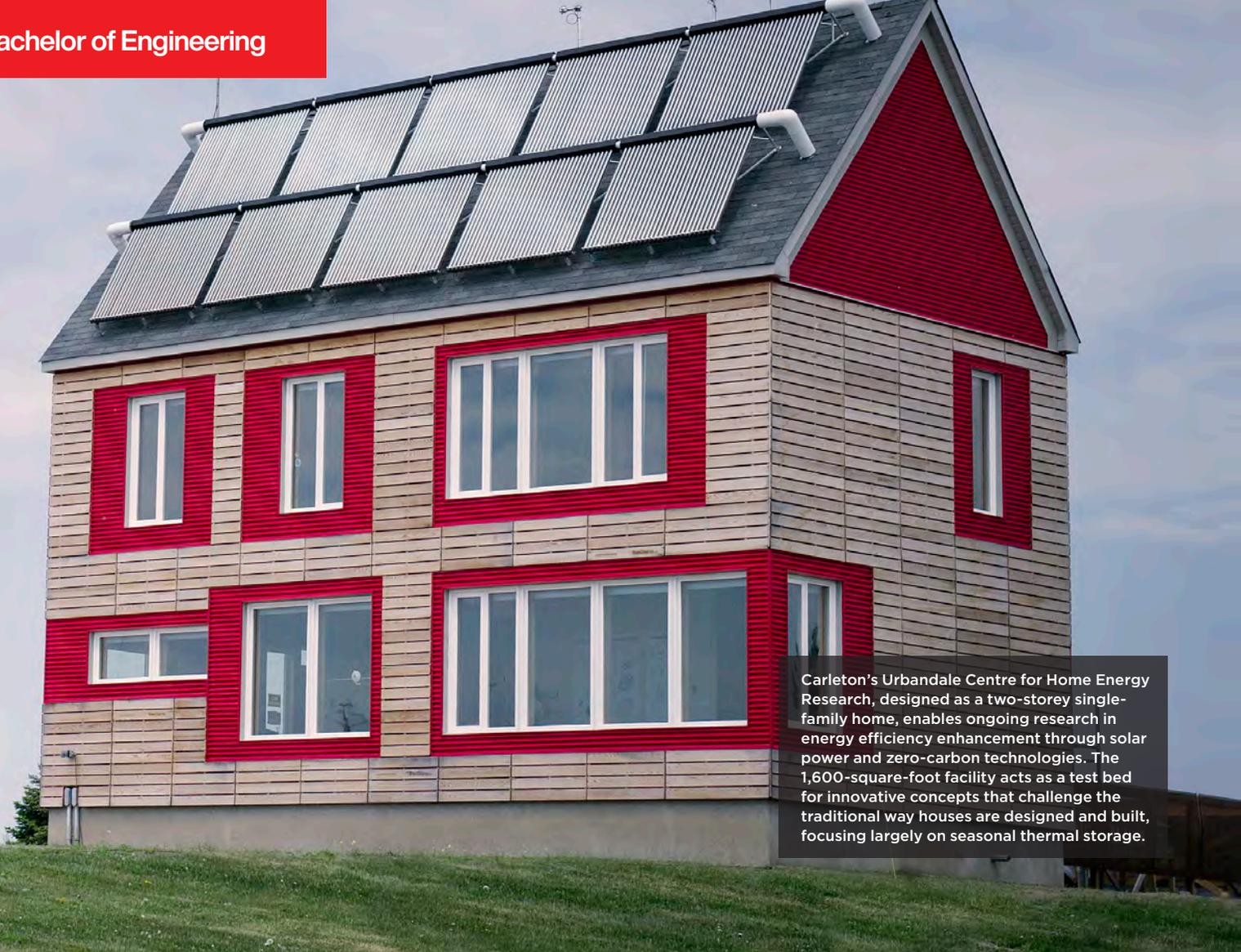
Carleton's Urbandale Centre for Home Energy Research, designed as a two-storey single-family home, enables ongoing research in energy efficiency enhancement through solar power and zero-carbon technologies. The 1,600-square-foot facility acts as a test bed for innovative concepts that challenge the traditional way houses are designed and built, focusing largely on seasonal thermal storage.
