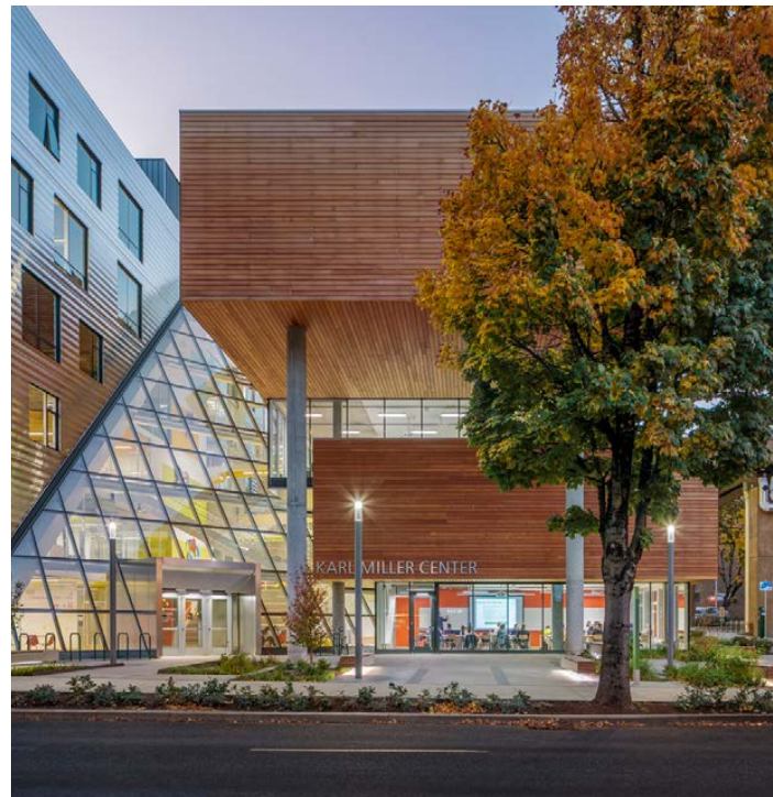
Buildings should utilize a variety of innovative and low-tech climate concepts to minimize environmental impact. (Karl Miller Center, Portland State University, USA, Behnisch Architekten, SRG Partnership © Brad Feinknopf)
