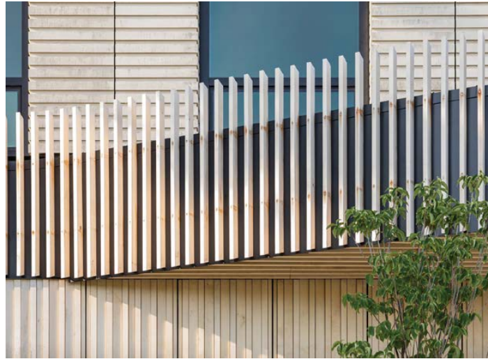
Mass timber building constructed at Oregon State University, Corvallis, USA (Oregon Forest Science Complex, Michael Green Architecture; ©Josh Partee)
