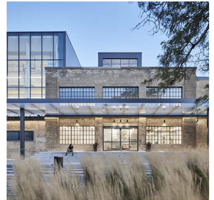
An example of an adaptive reuse project where a historic building was transformed into an innovation hub for Centennial College's Aviation and Engineering Technology program. (Centennial College; Toronto, Canada; MJMA in associated with Stantec Architecture Institutional © Doublespace Photography)
