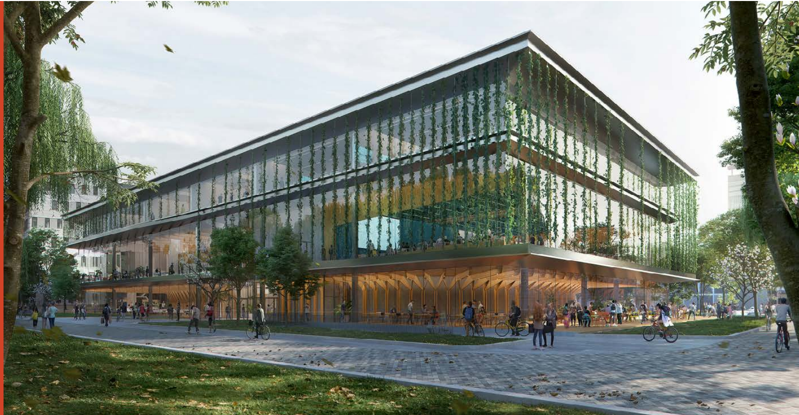
ECHO at Technical University of Delft was created as a future-proof, multi-functional and flexible inter-faculty building. Echo is centered on the adaptability and wellbeing of the user, programmed with a series of agile spaces that invite students and faculty to learn, collaborate and co-create. The building also harvests and produces more energy than it consumes. (Echo Energy-Generating Interfaculty Teaching Building, Delft, Netherlands, UNStudio © Plompmozes)
