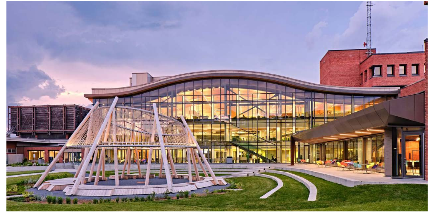
Landscape and building materials improve visibility in spaces, such as circulation corridors and stairwells, that may otherwise be narrow and isolated. (Algonquin College, Ottawa, Canada, Brook Mclroy; © Doublespace Photography)
