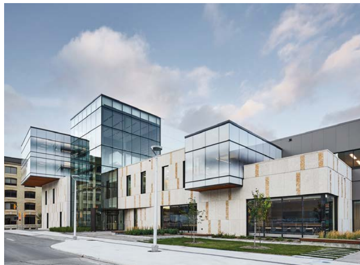
Building articulation and design assists in providing more natural daylight into the building. This also creates a strong urban edge and establishes a visual proportion, scale, and relationship to the street. (Laboratory Research Centre, Winnipeg, Number TEN Architectural Group © Stationpoint Photographic)
