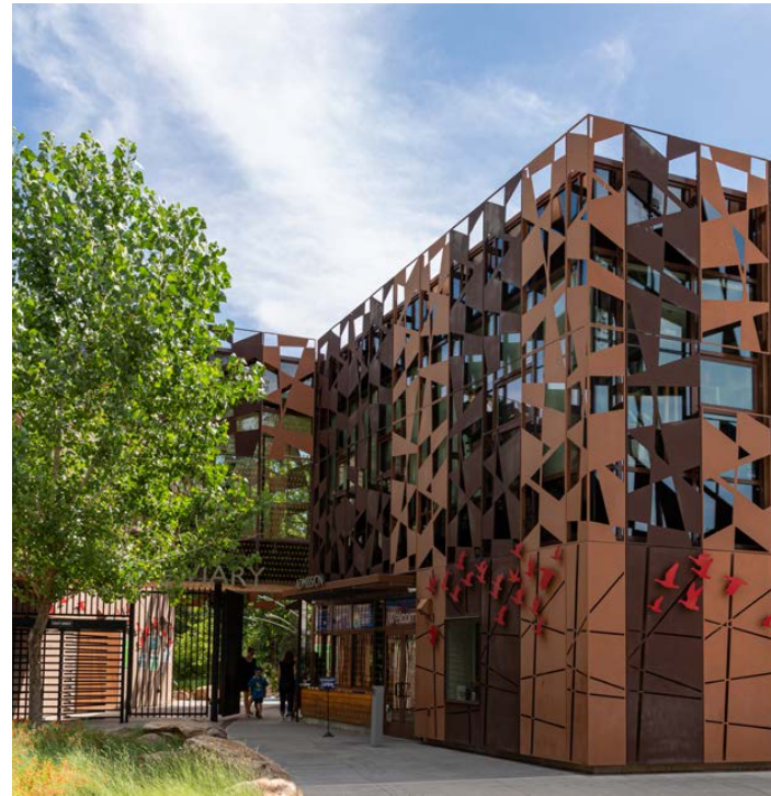
Using screens and opaque materials will reduce light pollution, sky glow, encourage a bird-friendly campus minimize energy demand and improve indoor thermal comfort. (Tracy Aviary, ajc architects ©Joseph Pollard)
