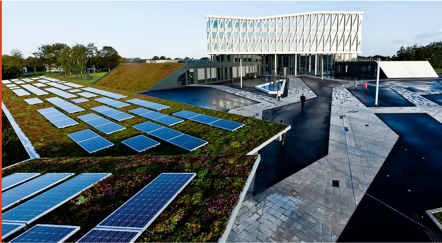
Green roof with solar panels. (Town and City Hall in Viborg, Denmark, Henning Larsen© Thorbjorn Hansen)
