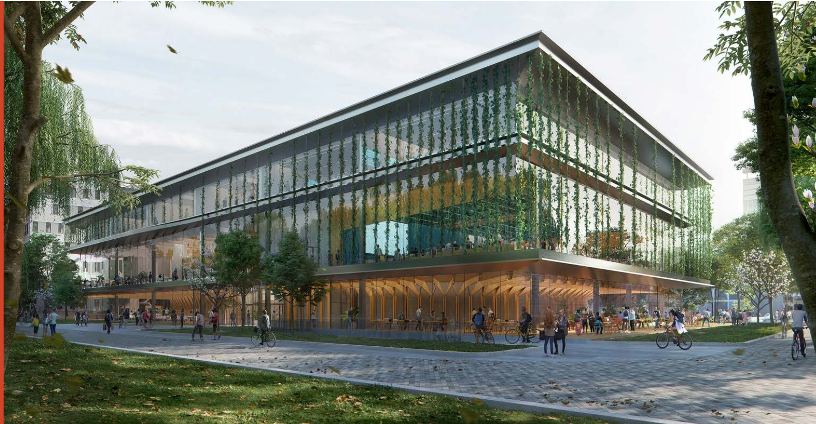
ECHO at Technical University of Delft was created as a future-proof, multi-functional and flexible inter-faculty building. Echo is centered on the adaptability and wellbeing of the user, programmed with a series of agile spaces that invite students and faculty to learn, collaborate and co-create. The building also harvests and produces more energy than it consumes. (Echo Energy-Generating Interfaculty Teaching Building, Delft, Netherlands, UNStudio © Plompmpozes)
