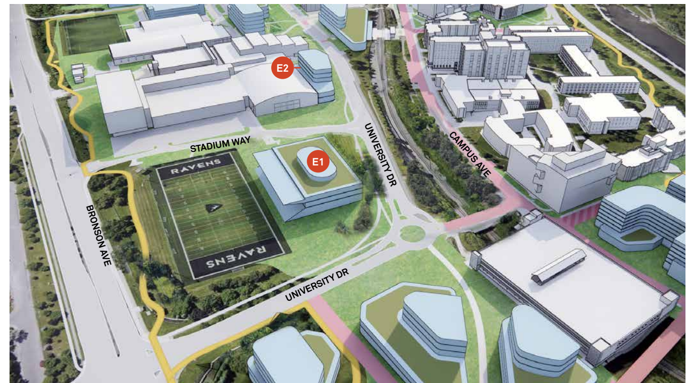
Site E1 and E2. View looking southwest.
