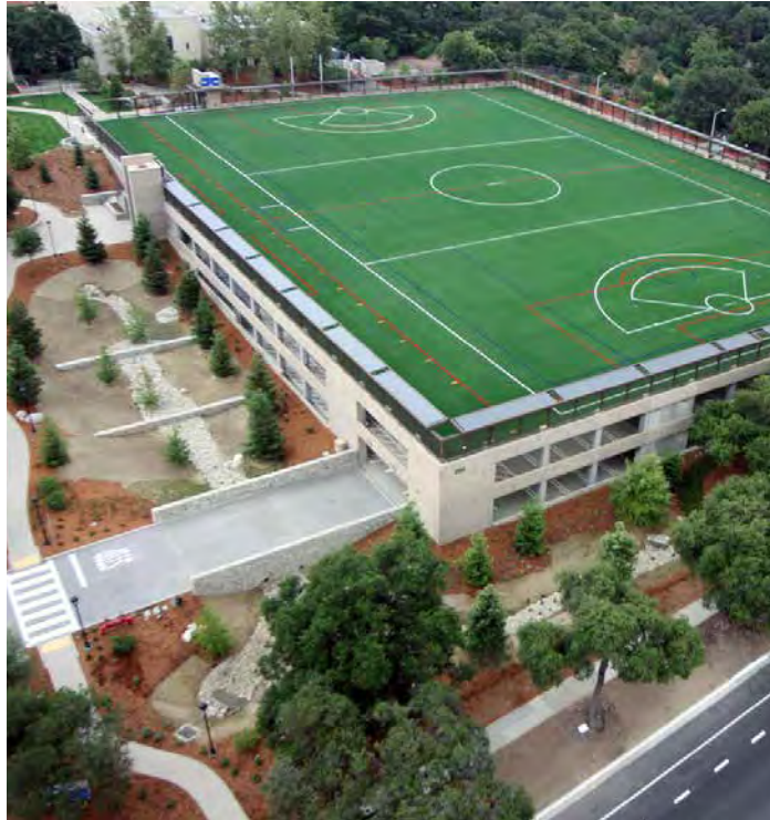
Example of a multi-use parking structure with a rooftop synthetic turf sport field that reduces irrigation by 50,000 gallons of water per week, filters water, and reduces discharge into the environment. (Claremont, CA. Watry Design, Inc. © Pomona College)
