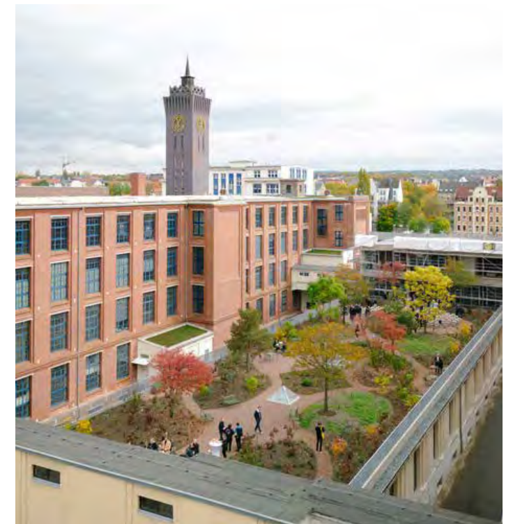
Rooftop gardens and greenroofs can be used for outdoor meetings, lectures, and events. Green roofs not only retain water but can act as natural filters for water runoff and can decrease stress on sewer systems at peak flow periods. (Chemnitz, Germany, Meyer-Grohbrügge © Johannes Richter)
