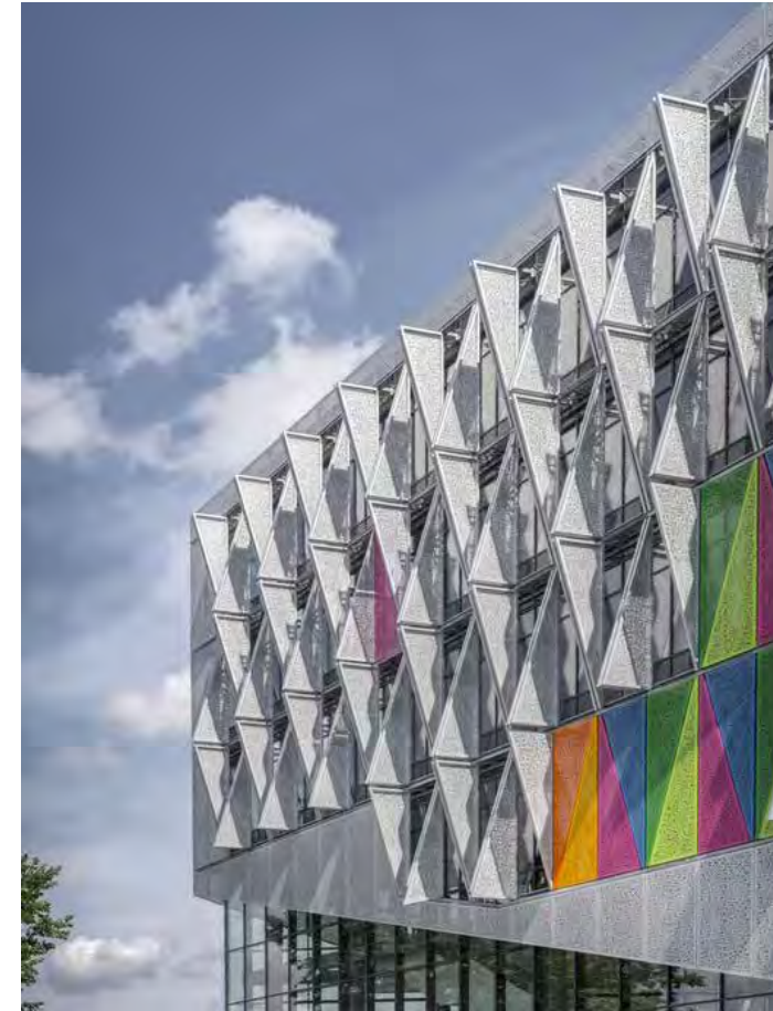
Dynamic solar shading systems mounted on the façade can adjust to the specific climate conditions, user patterns and provide optimal daylight. (SDU Campus, Henning Larsen © Martin Schubert)
