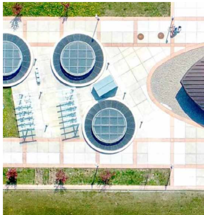
Westbrook LRT Station, Calgary. (© GEC Architecture)
