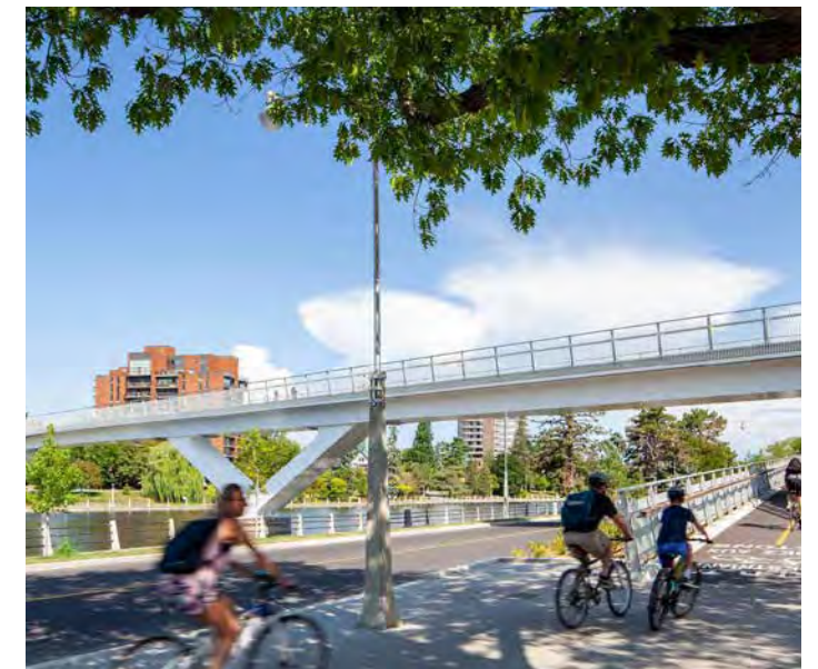
Promote active forms of transportation through infrastructure (Flora Footbridge, Ottawa, Canada © DTAH)
