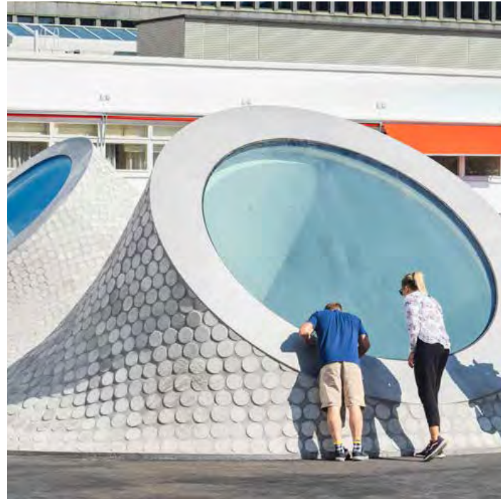
Skylights integrated into public spaces. (Amos Rex, a below-grade art museum, Helsinki, JKMM © Mika Huisman)
