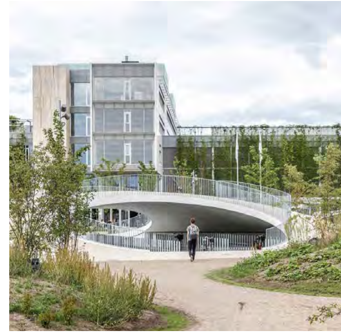
Karen Blixens Plads is an undulating plaza that mimics the surrounding landscape and provides sheltered parking for over 2,000 bicycles for the university's students and staff. (Karen Blixens Plads, Copenhagen, COBE & COAST © Rasmus Hjorthøj)
