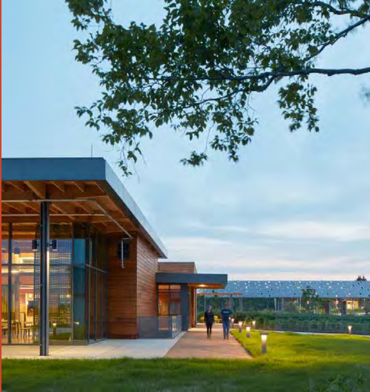
The Chatham University Eden Hall Campus generates more energy than it uses, produces food, recycles nutrients, and supports habitat and healthy soils. (Pennsylvania, Mithun © Bruce Damonte)
