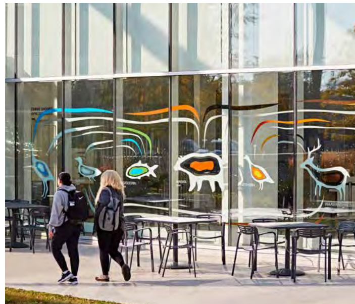
Window markings can incorporate Indigenous design and aid in wayfinding. (© Brook McIlroy)
