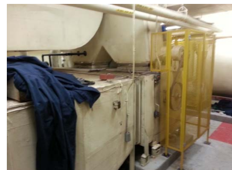
Typical Air Handling Unit
