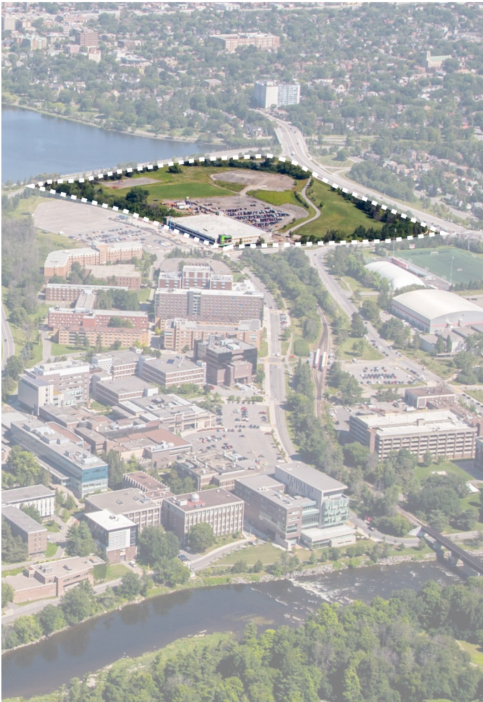
Existing aerial image highlighting the north campus area
