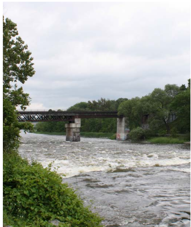
Existing naturalized buffer along the banks of the Ottawa River
