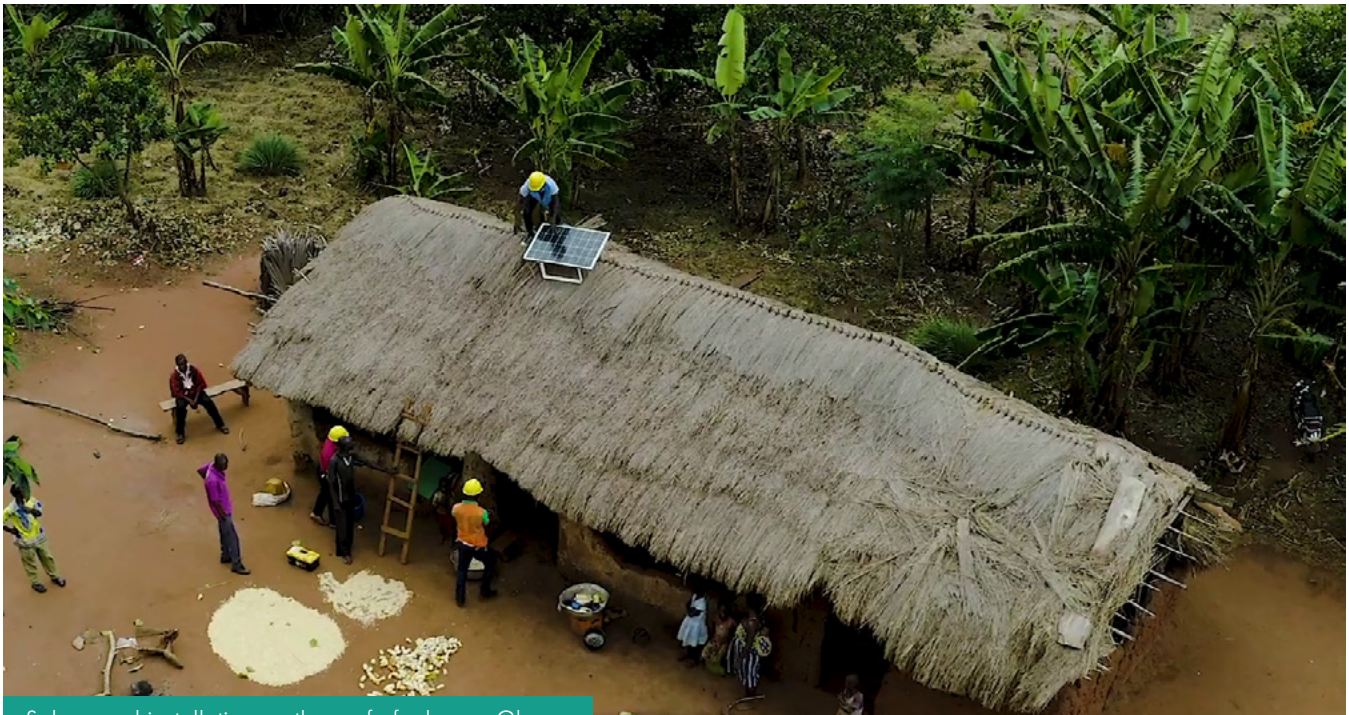
Solar panel installation on the roof of a home, Ghana.
