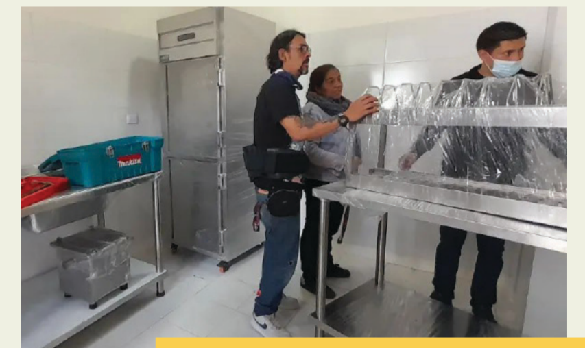
Kitchen appliances being installed in the community kitchen.
