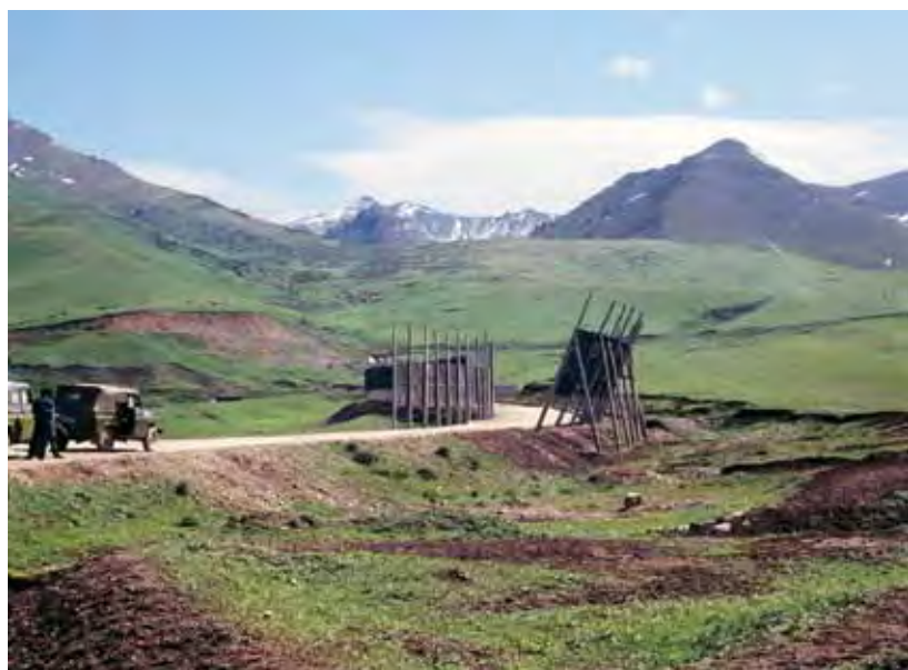
Fig. 60. Well above the timberline in the central Tian Shan we inspect the famous baffles erected to combat heavy drifting snow across the open tundra.
