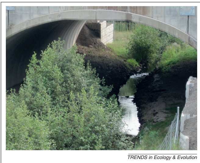
Figure 1. Example of an ‘extended stream crossing’ over a stream in New Brunswick, Canada. Design details will vary but the width of the extended stream crossing should be approximately five times the width of the stream at high water, allowing dry passage of terrestrial animals along its banks. The height should be sufficient to allow passage of the tallest animal for which mitigation is desired, here moose, Alces alces . Reproduced, with permission, from L. Fahrig.
