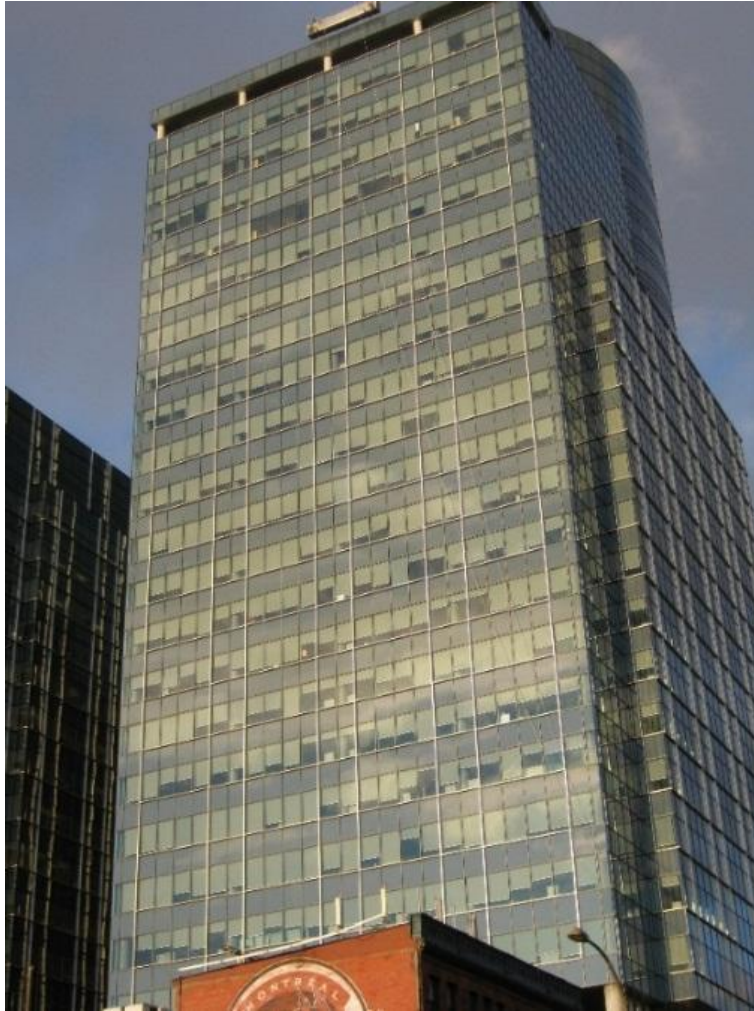
Figure 10. Typical modern building design: highly-glazed facades (O'Brien and Gunay, 2015).
