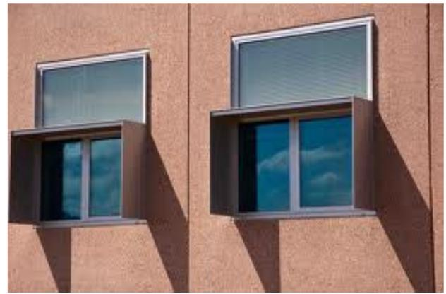
**Figure 5:** Exterior of NREL RSF space showing fixed shading (lower portion) and light louvers (upper portion).
