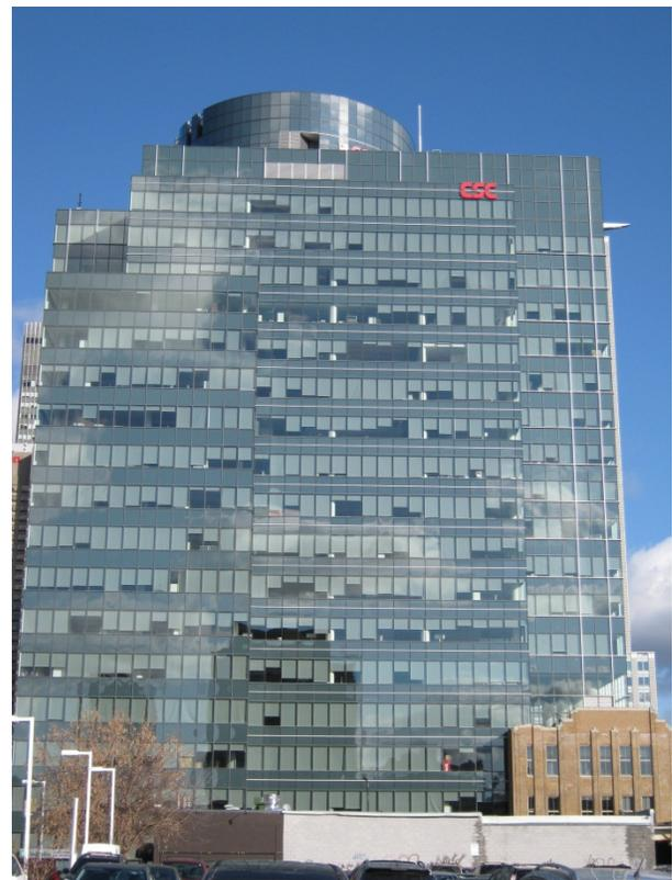
**Figure 2:** Typical shade deployment levels of a south-west facing office building façade in the winter.
