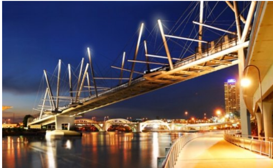
Figure 1.3: Tensegrity Bridge: The Kurilpa Bridge is a tensegrity structure that spans the Brisbane River in Brisbane, Australia [10].
