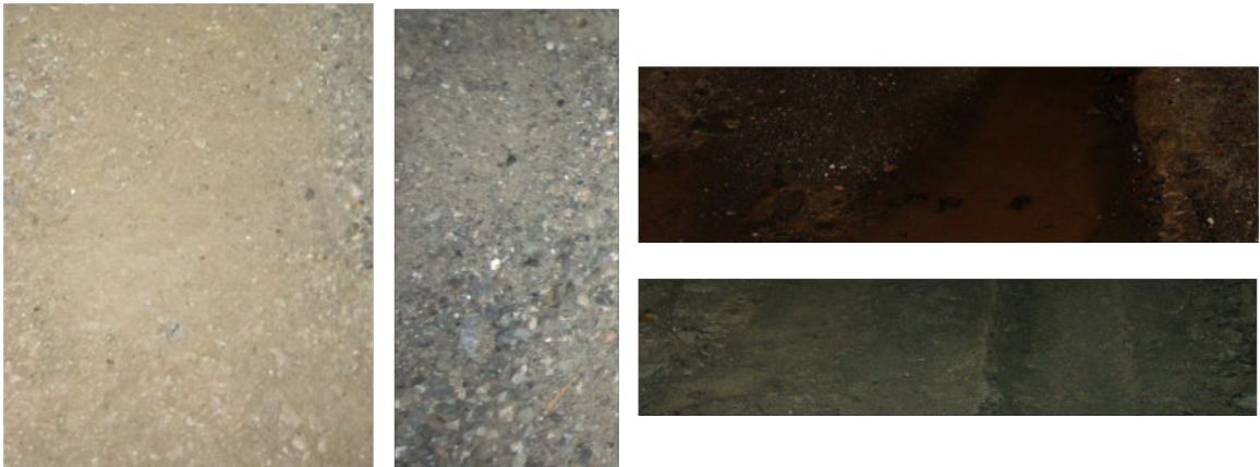
Figure 3.12: CANMET Tunnel Floor Textures.
