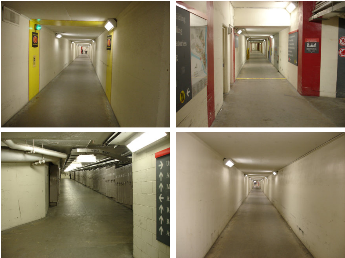
Figure 4.4: Photos of the CU underground tunnels.
