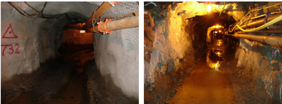
Figure 4.5: CANMET Experimental Mine tunnel photos.
