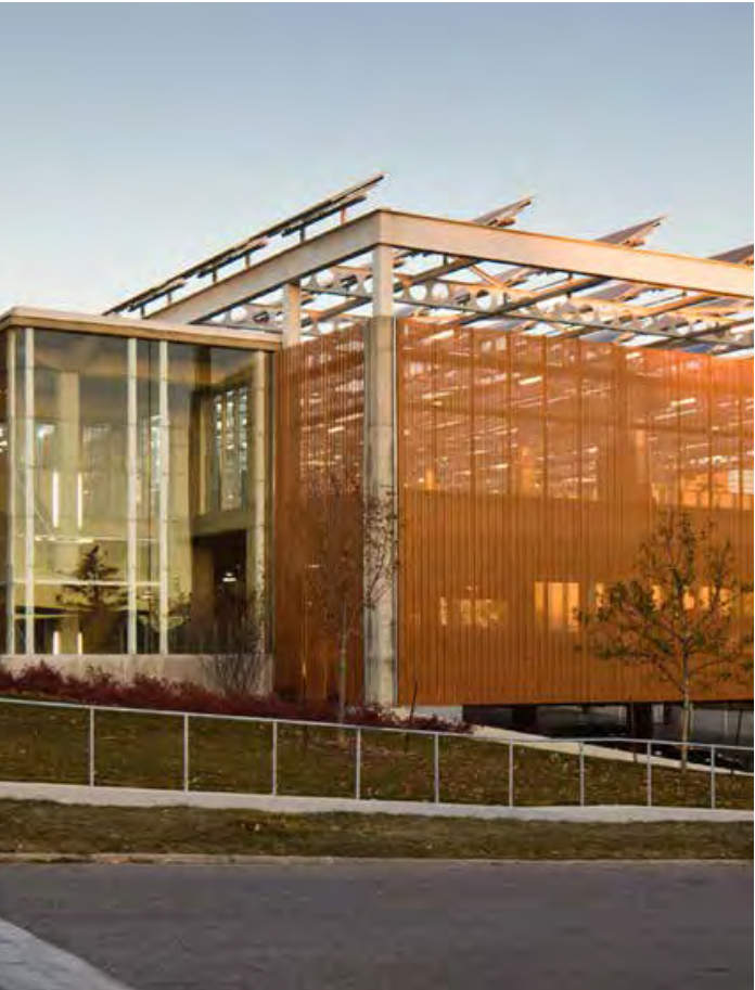
Example of a parking garage with passenger shelters with a solar panel array on the roof to produce a net-zero electricity use for the building. (The University of Northern Iowa’s Multi-modal Transportation Center, United States, Substance Architecture © Paul Crosby Architectural Photography)
