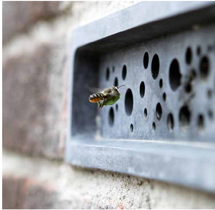
Building materials can safely incorporate habitats for bees, birds, and bats. The pictured Bee Brick replaces a brick in the wall and provides a nesting place for solitary bees within the irregular pattern of holes. (© Green & Blue)
