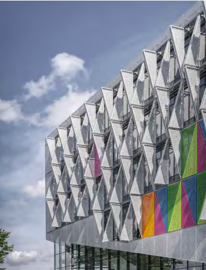
Dynamic solar shading systems mounted on the façade can adjust to the specific climate conditions, user patterns and provide optimal daylight. (Southern Denmark University Campus, Henning Larsen© Martin Schubert)
