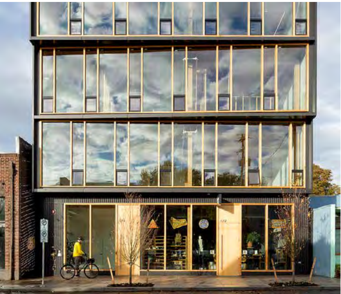
An example of mass timber construction with a glue-laminated timber frame and Cross-Laminated Timber panels. (Portland, USA; LEVER ©Jeremy Bitterman)
