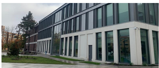
Carleton's new Engineering Design Centre provides flexible labs and collaboration space
