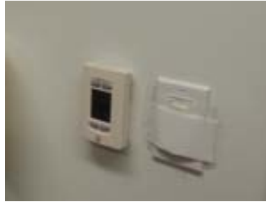
Figure 2.1: An example where the occupant taped over the motion detectors (credit: Sara Gilani).
