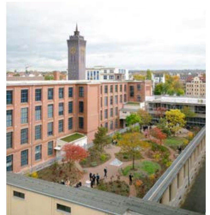
Rooftop gardens and greenroofs can be used for outdoor meetings, lectures, and events. Green roofs not only retain water but can act as natural filters for water runoff and can decrease stress on sewer systems at peak flow periods. (Chemnitz, Germany, Meyer-Grohbrügge © Johannes Richter)
