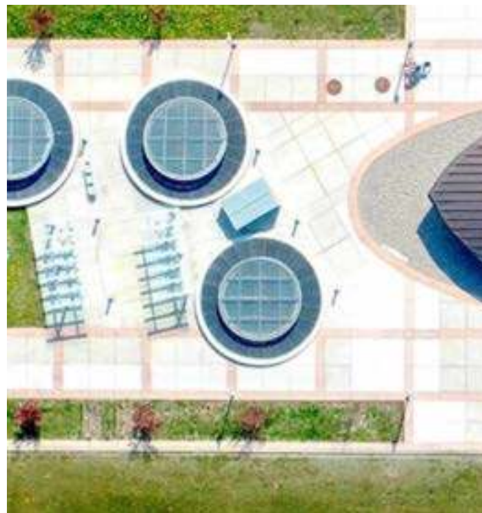
Westbrook LRT Station, Calgary. (© GEC Architecture)
