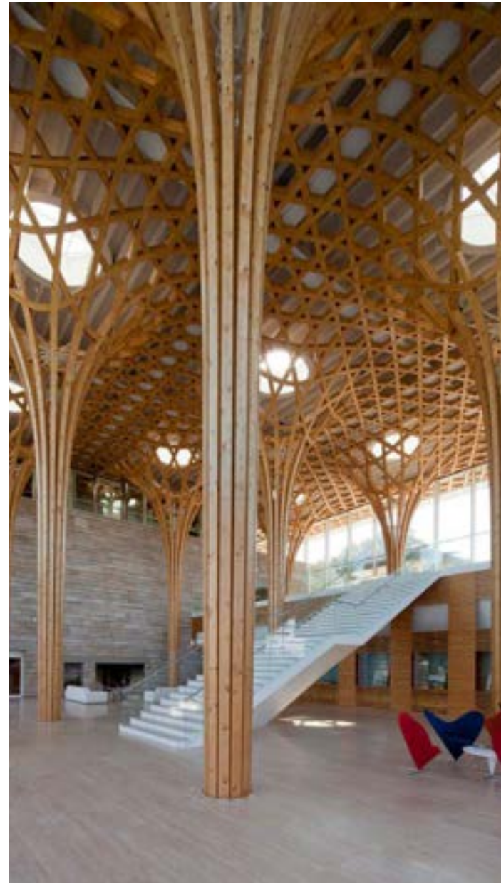
Example of enclosed atrium designed with tree-like columns and natural material cladding to evoke a sense of the outdoors. (Nine Bridges Country Club, Shiguru Ban Architects © Hiroyuki Hiarai)
