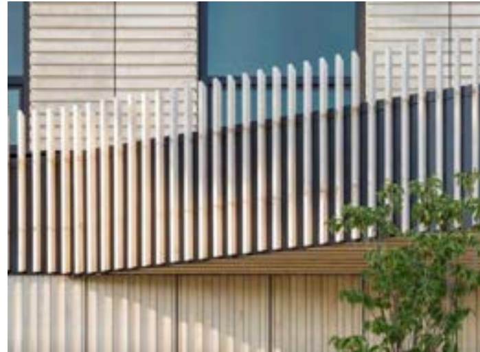
Mass timber building constructed at Oregon State University, Corvallis, USA (Oregon Forest Science Complex, Michael Green Architecture; ©Josh Partee)
