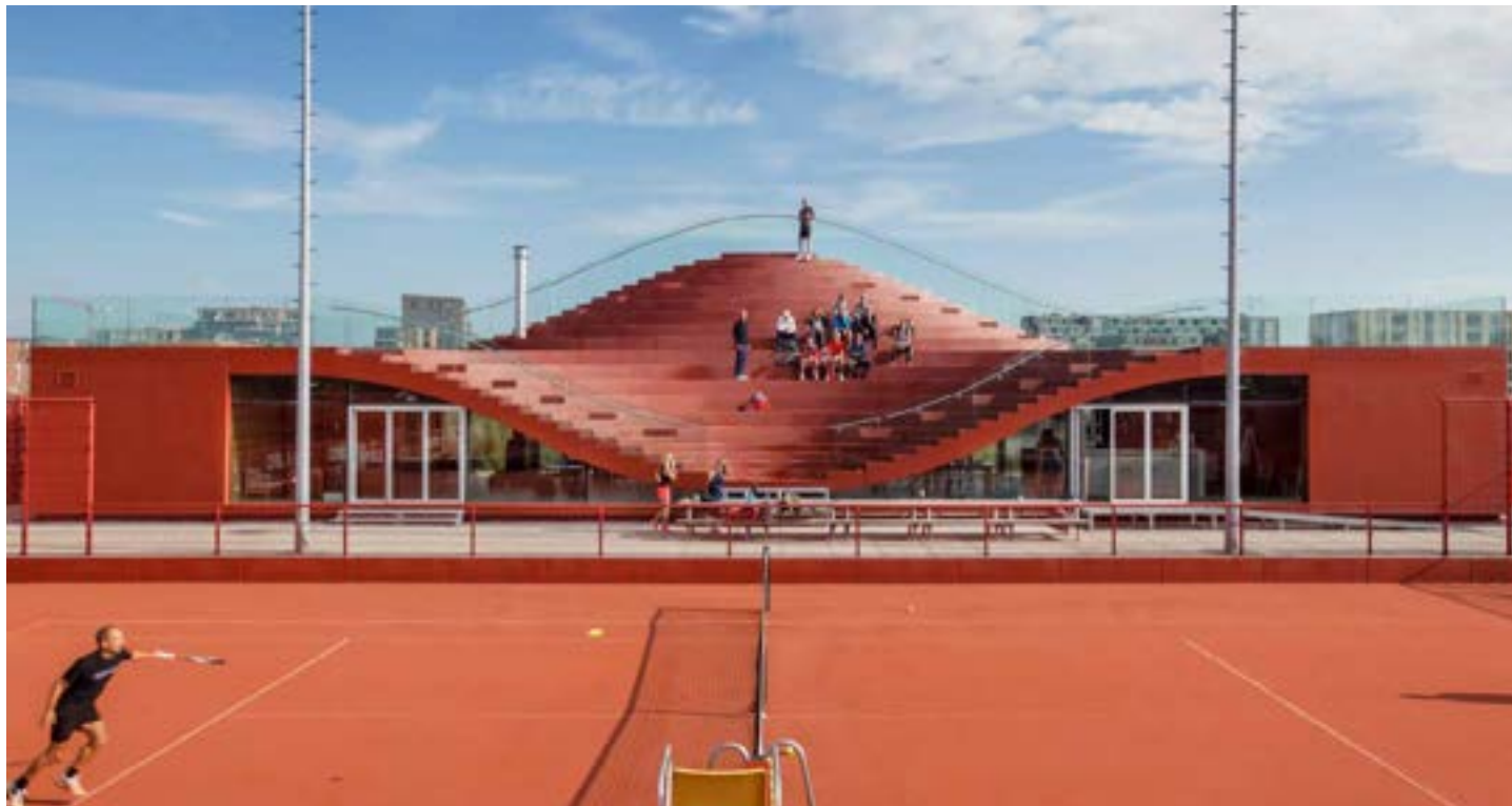
The image above shows a bright red tennis clubhouse which acts as an advert for sports and movement. The rooftop also doubles as an expansive seating area for game spectators. Housed inside the structure are utility areas, changing rooms, and kitchen facilities. (Amsterdam Tennis Clubhouse, Netherlands © MVRDV)
