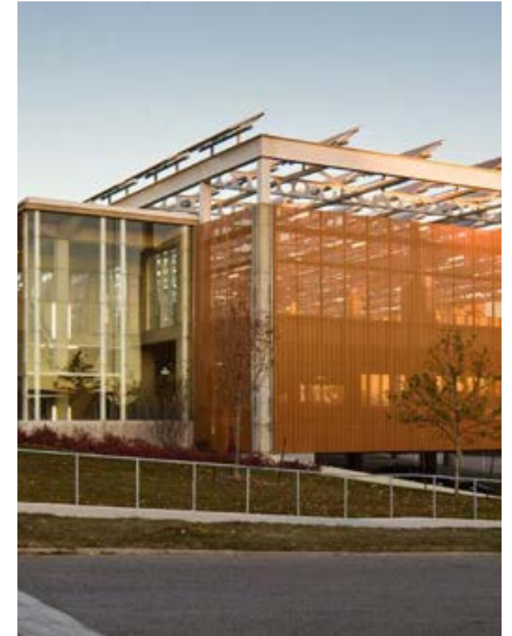
Example of a parking garage with passenger shelters with a solar panel array on the roof to produce a net-zero electricity use for the building. (The University of Northern Iowa’s Multimodal Transportation Center, United States, Substance Architecture © Paul Crosby Architectural Photography)
