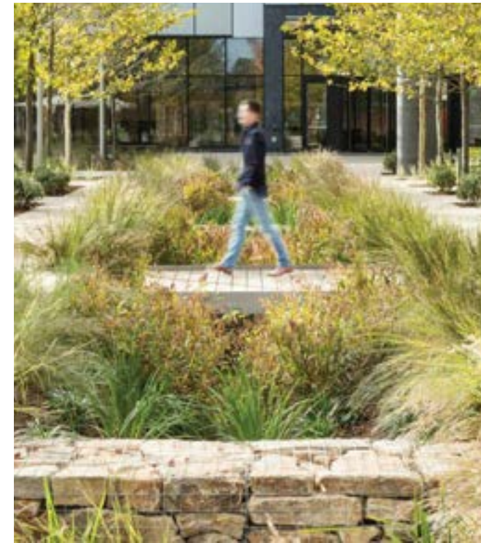
Rain gardens collect stormwater runoff and are often planted with native species that do not require permanent irrigation. (Somerville, Massachusetts, OJB © Kyle Cadwell)
