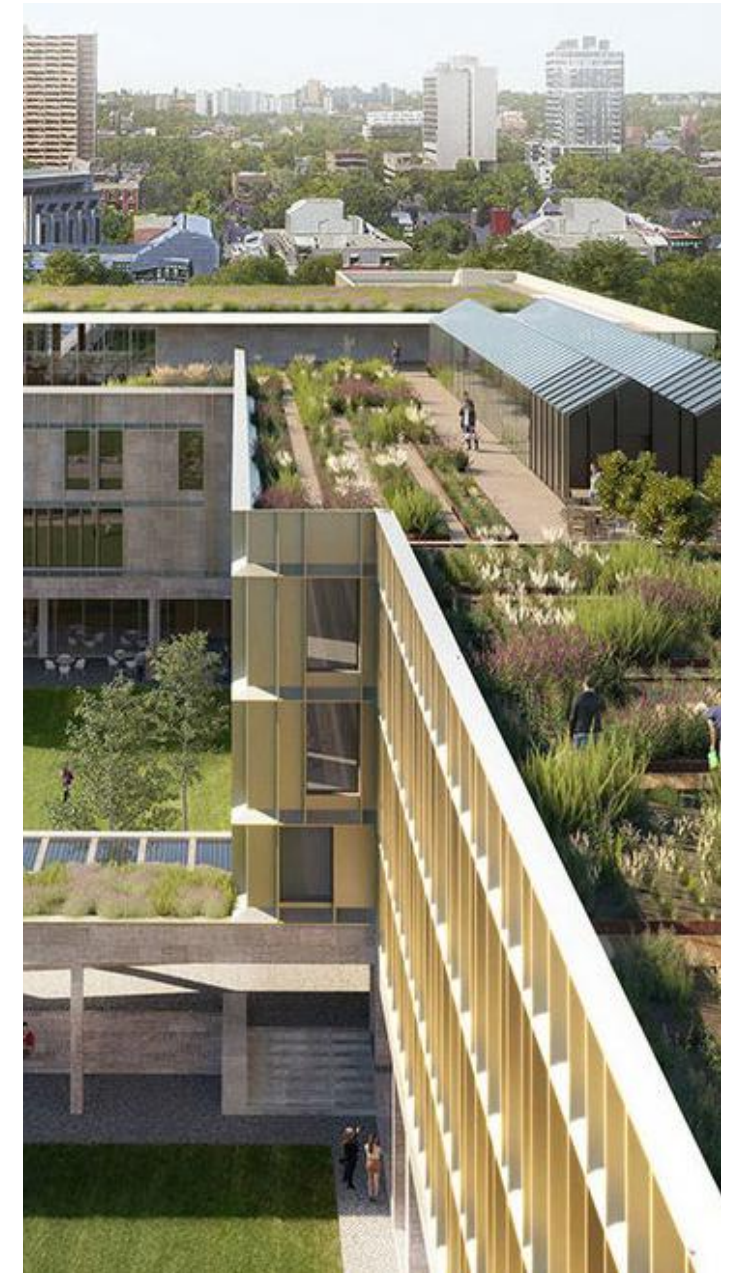
Green roofs offer many environmental and human health benefits such as air purification, increased biodiversity, reduced building energy costs and urban heat island amelioration, and stormwater runoff mitigation. (Lawson Centre for Sustainability, Trinity College, University of Toronto ©RHDA and Mecanoo Architecten)
