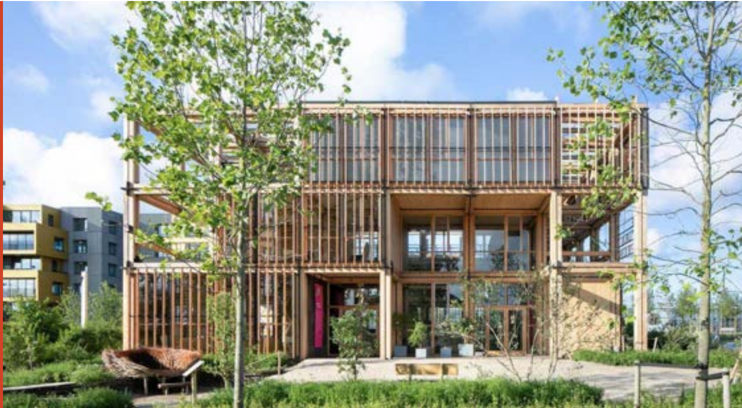
The Natural Pavilion showcases innovative bio-based construction and circular design that can be easily disassembled and rebuilt in a different configuration at a different location. (The Natural Pavilion, Netherlands, DP6 architectuurstudio © Daria Scagliola & Stijn Brakkee)
