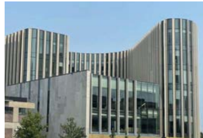
Nicol Building at Carleton University. (Hariri Pontarini Architects © Brook McIlroy)
