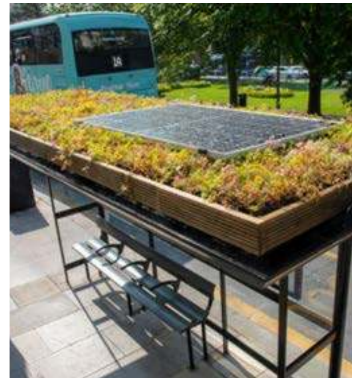
Solar-powered shelters with a living roof planted with a mix of wildflowers helps support biodiversity, provides a resting stop for pollinators, absorbs rainwater and is powered by solar energy. The bus stop is also designed with principles of circular economy. (Bee Bus Stop, ©Brighton & Hove City Council)
