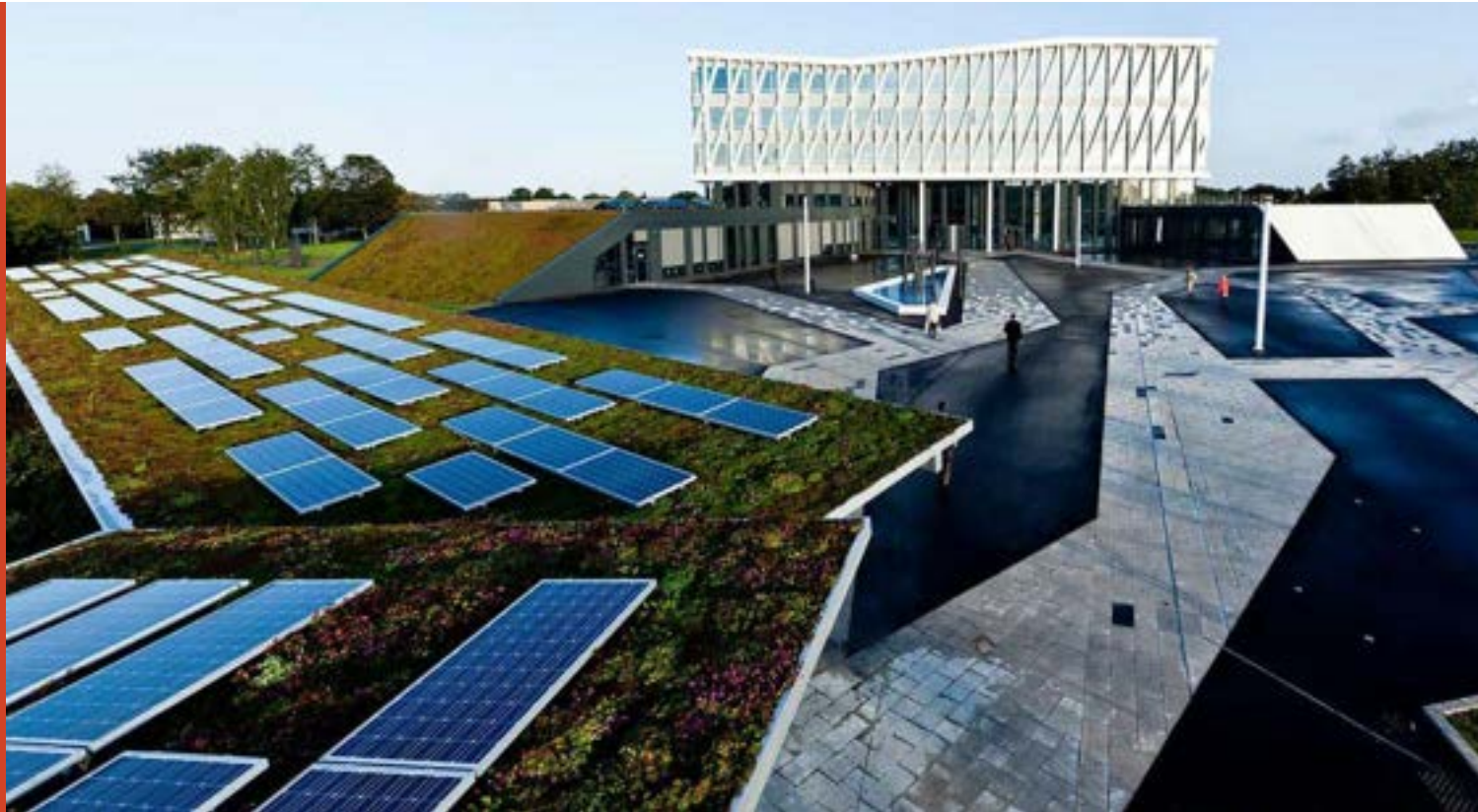
Green roof with solar panels. (Town and City Hall in Viborg, Denmark, Henning Larsen© Thorbjorn Hansen)
