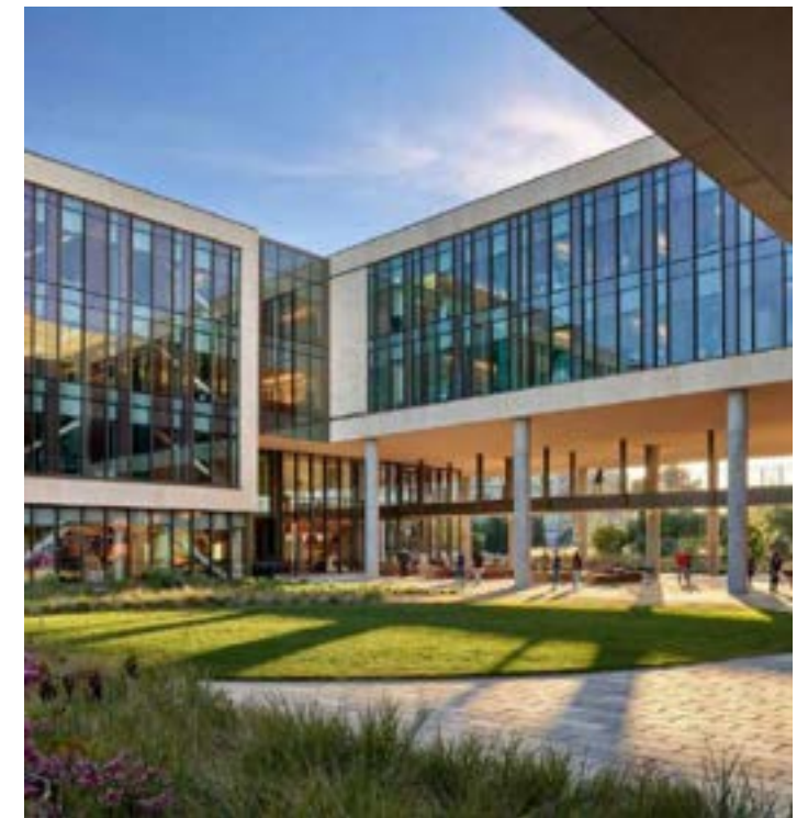
A passive-first design approach takes full advantage of the site while reducing energy consumption. The sun, wind, and ecosystem can influence everything from the initial planning decisions to the building details. (Stanford University School of Medicine Center for Academic Medicine; HOK © Alan Karchmer)
