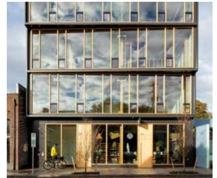
An example of mass timber construction with a glue-laminated timber frame and CLT panels. (Portland, USA; LEVER ©Jeremy Bitterman)
