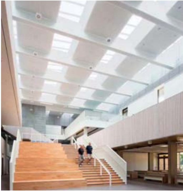
Designed to provide daylight and fresh air through the roof, VELUX Modular Skylights help create healthy, comfortable and productive indoor spaces. The modular system can be configured to a range of different skylight solutions and offers several features for climate control, ventilation, and shading. (Trumpington Community College, Great Britain ©VELUX)
