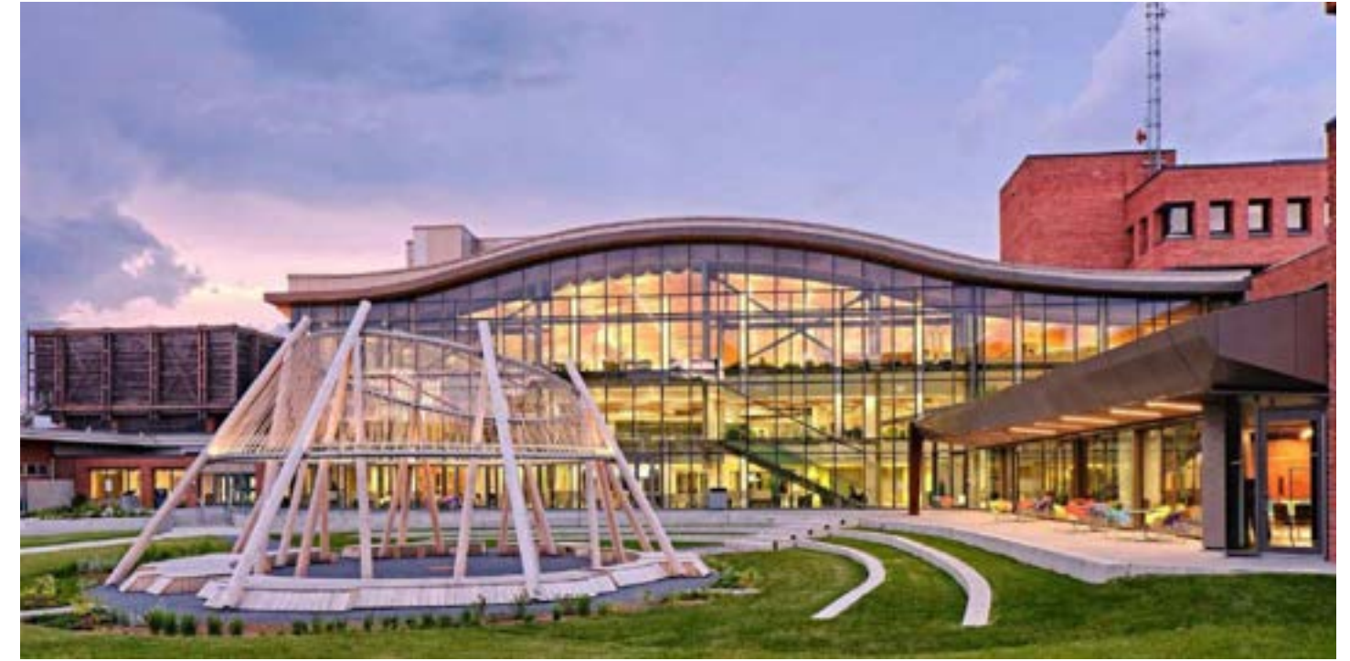
Landscape and building materials improve visibility in spaces, such as circulation corridors and stairwells, that may otherwise be narrow and isolated. (Algonquin College, Ottawa, Canada, Brook McIlroy; © Doublespace Photography)
