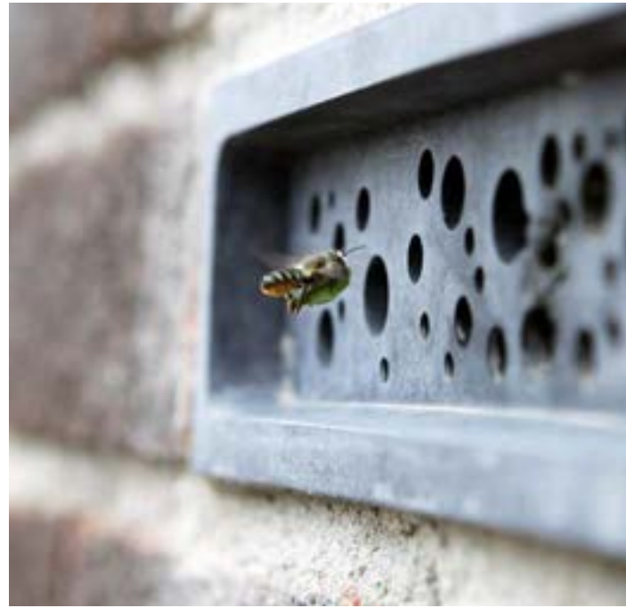
Building materials can safely incorporate habitats for bees, birds, and bats. The pictured Bee Brick replace a brick in the wall and provides a nesting place for solitary bees within the irregular pattern of holes. (© Green & Blue)
