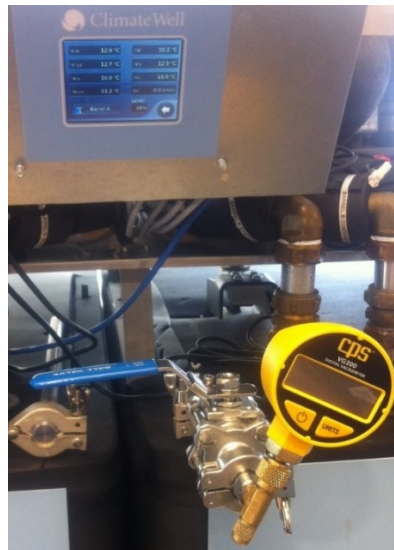
Figure 3-6: Modified evacuation set-up
