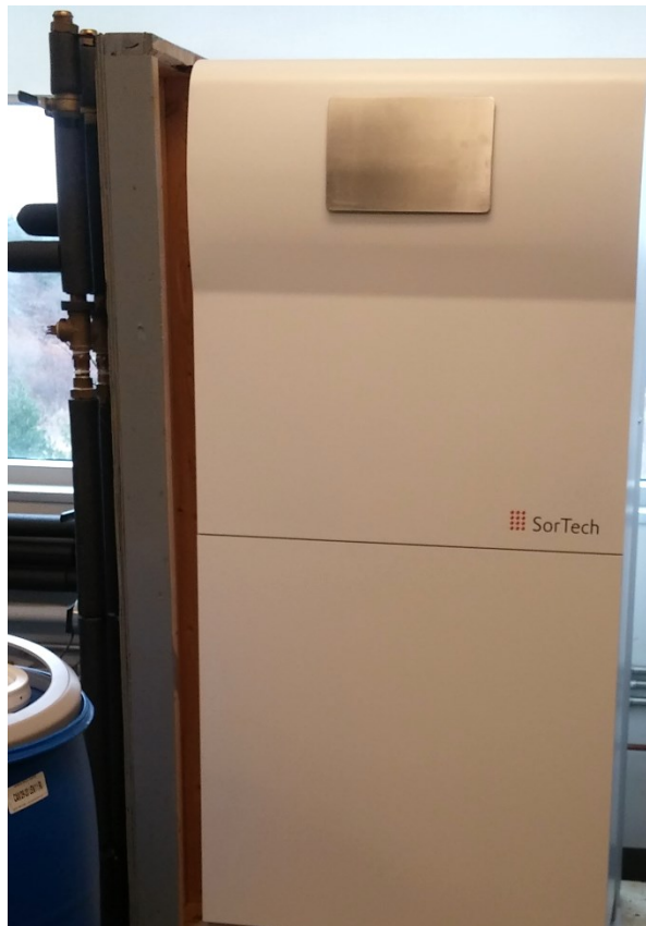
Figure 6-1: Recently acquired SorTech eCoo 2.0 adsorption chiller
