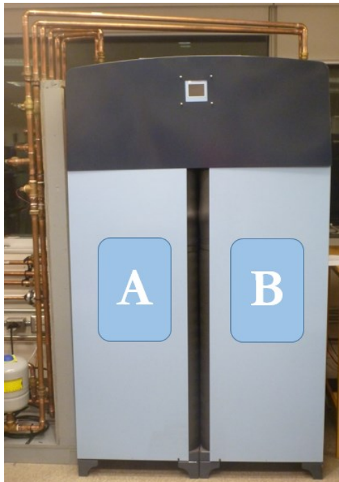
Figure 3-2: ClimateWell sorption chiller installed within the lab
