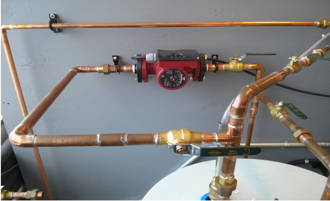
Figure 3-6: Anti-Stratification Pump
