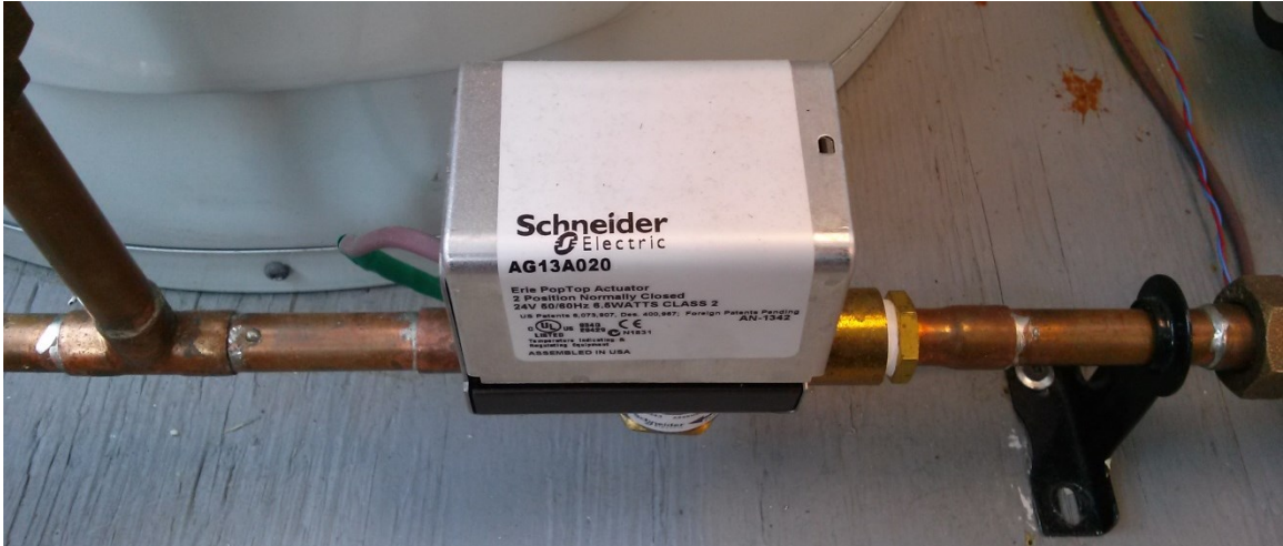
Figure 3-7: Normally Closed Solenoid Valve for Draw Profile Control
