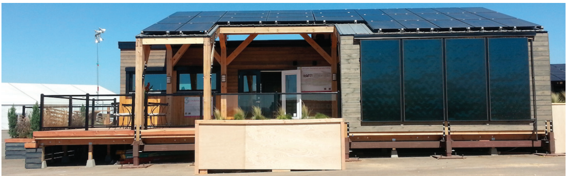
Figure 1.8: South side of ECHO with exo-structure holding photovoltaic panels on top and solar collectors on the front (Photo credit: Jacob Morgan)
