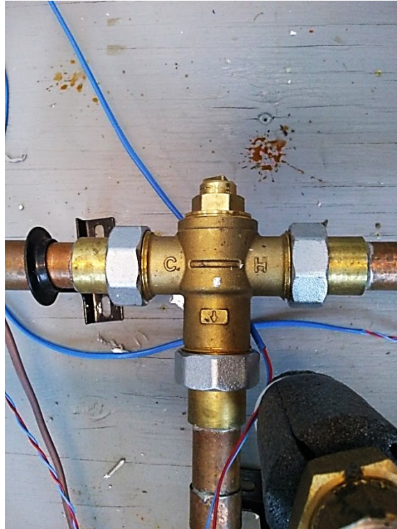
Figure 3-12: Tempering valve
