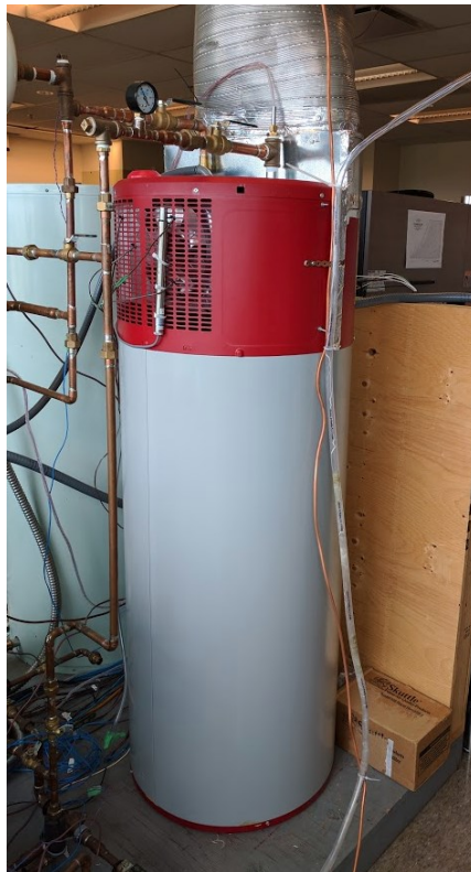
Figure 3-6: Heat pump water heater
