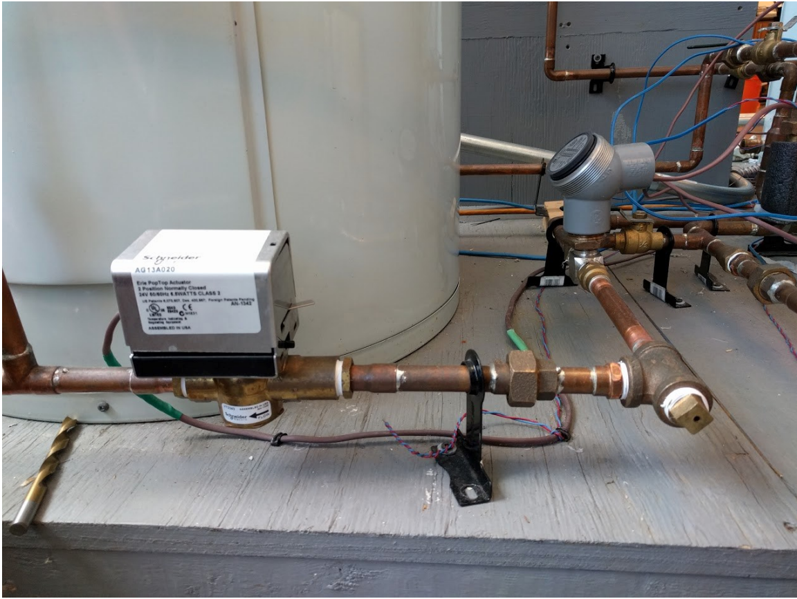
Figure 3-5: Water draw system, with the solenoid on the left and the water flow meter on the right
