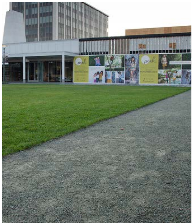
Stabilized decomposed granite
