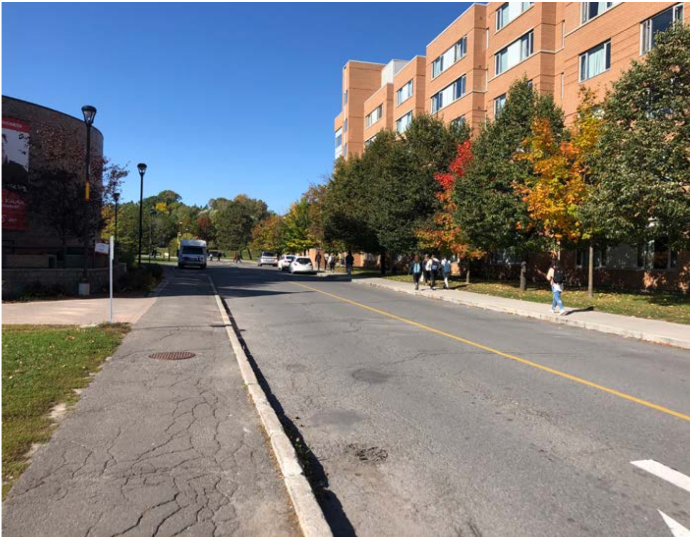
Existing Condition, Library Road (North)
