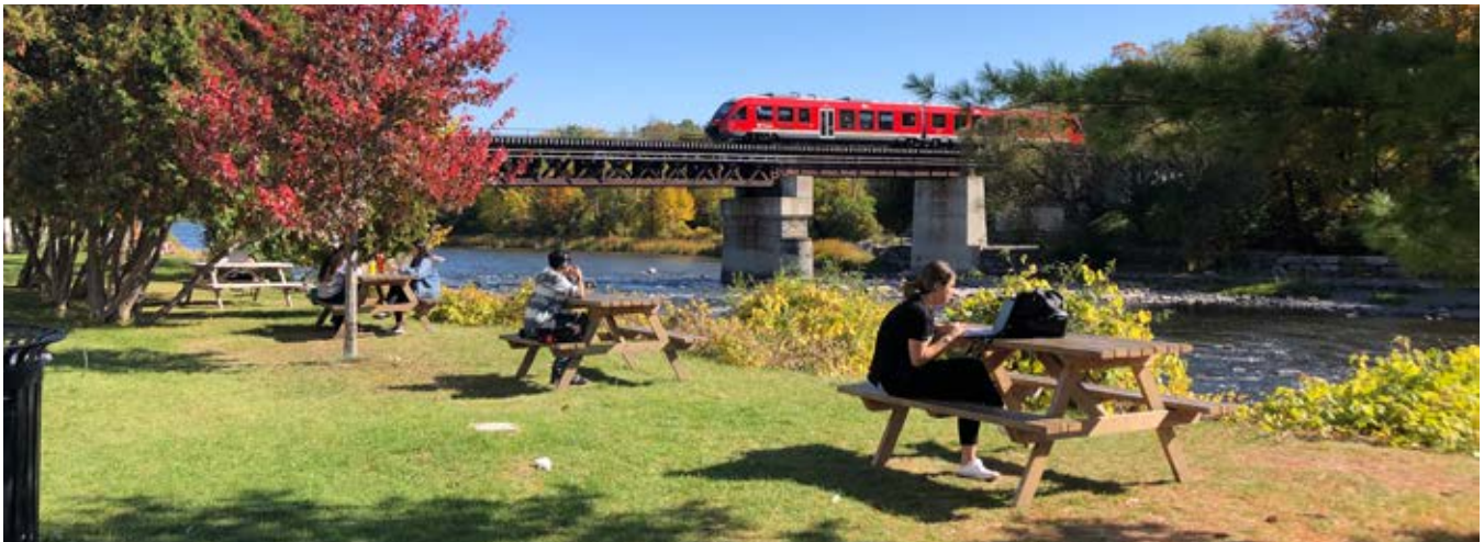
The O-Train Bridge across the Rideau River
