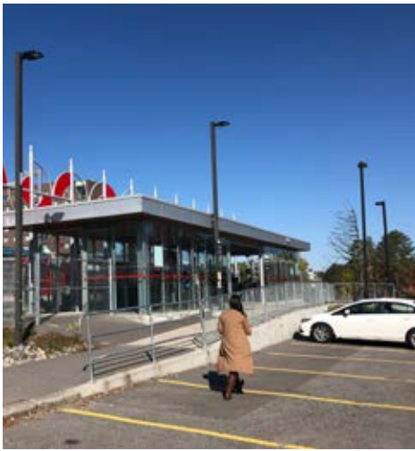
Eastern O-Train Station
