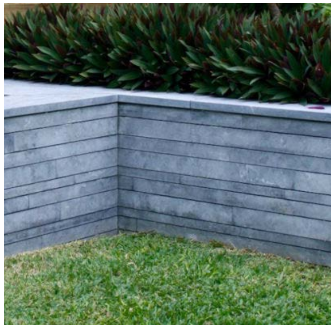
Limestone veneer retaining wall
