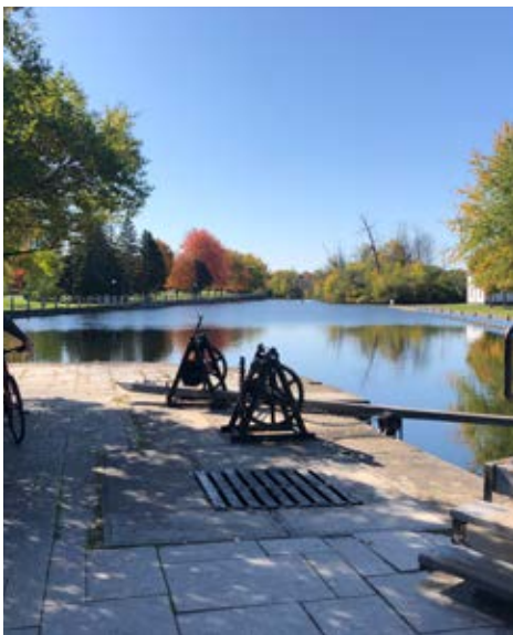
Crossing at the Hartwell Locks
