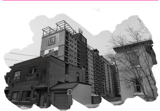
Before the apartment complex at 207 Bell Street North was transformed into a luxury condo-style apartment building, it served as a de facto housing resource for low- and middle-income households in West Centretown. The pre-renovation Bell Terrace building offered 1-bedroom unit rents of between $750 - $900 per month (all utilities included).
