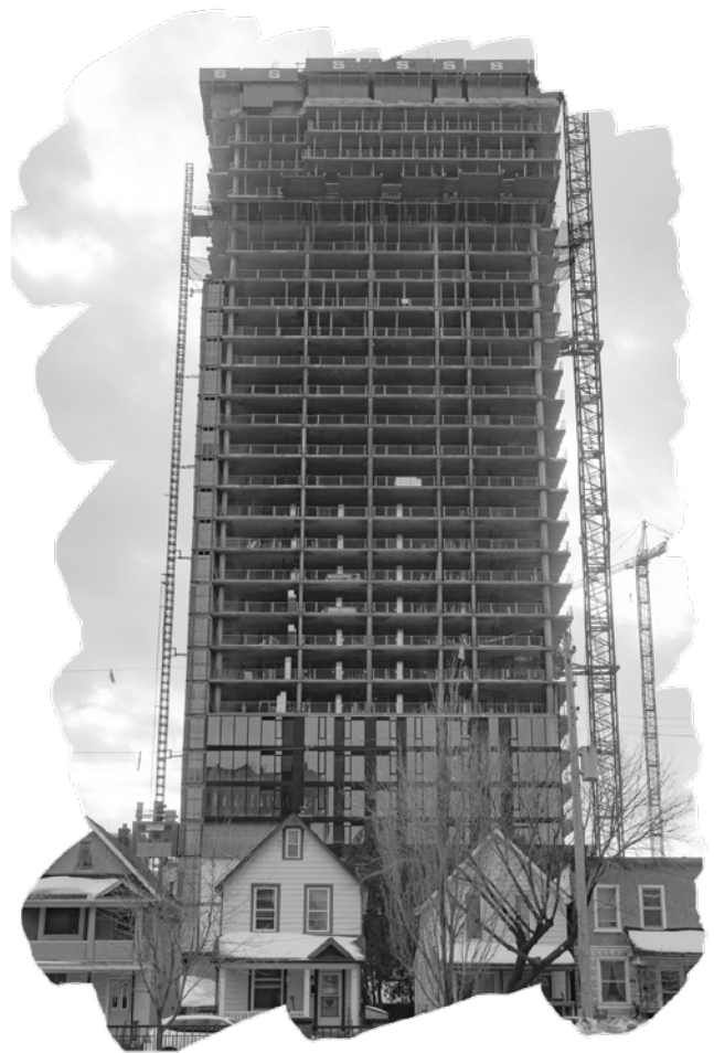
Figure 1. West Centretown is in the midst of development boom
